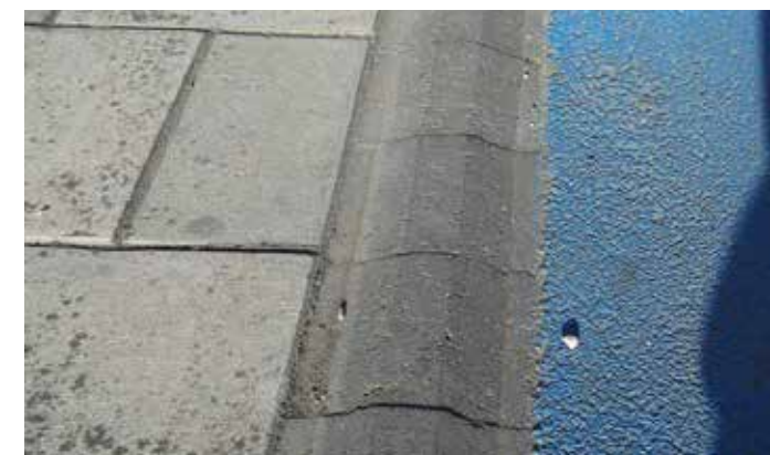
200mm demarcation kerb between footway and cycleway.
