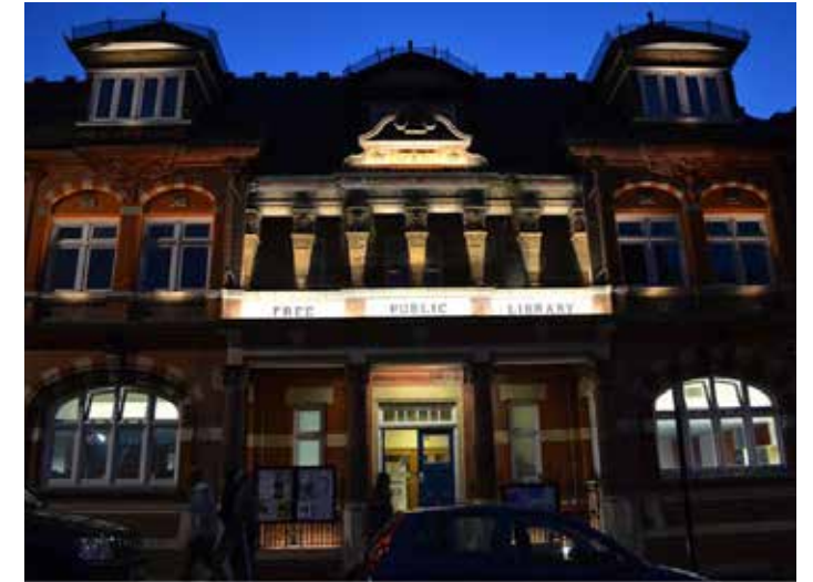
Architectural lighting focused on highlighting key architectural features ©Studio Dekka
