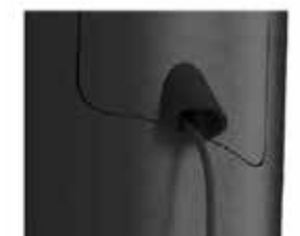
Secondary door for power supply with drip cover for cable
