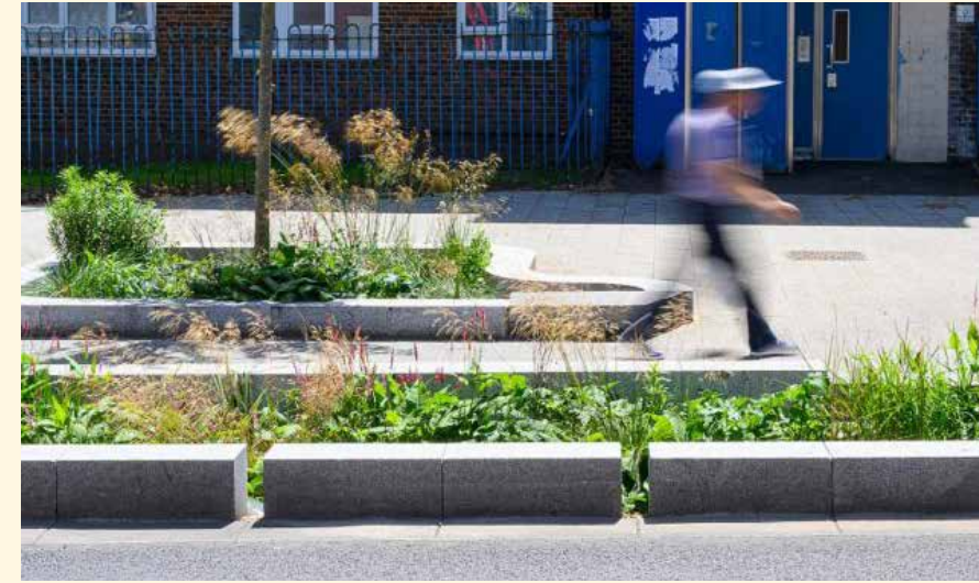
Example of rain gardens with a upstanding kerb edge. ©Robert Bray Associates
