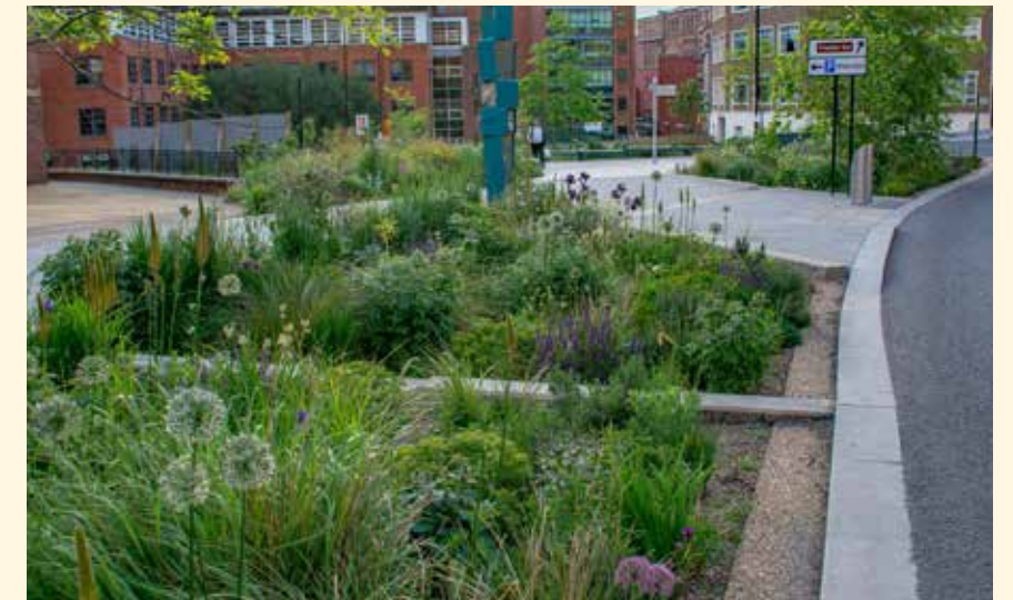
Large rain garden with check dams to control peak rainfall on a slope. ©Nigel Dunnett
