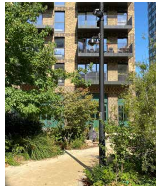
CCTV cameras in Elephant Park, London are mounted to low level light columns and adjacent to significant tree planting and low level planting
