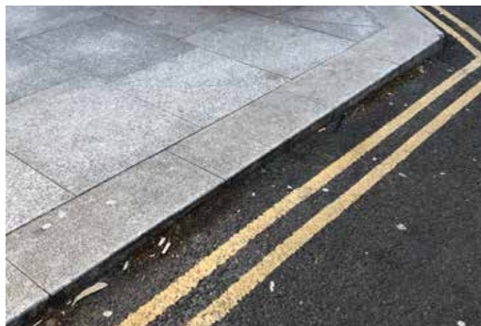
Kerb with low upstand height to encourage informal pedestrian crossing along a street
