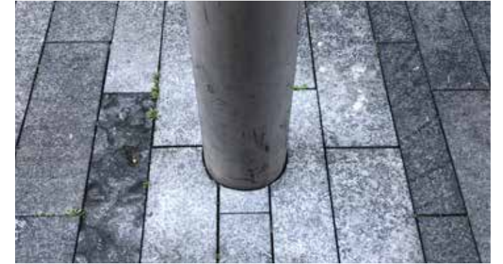
Paving should be cut with precision to ensure high quality. Cuts should reduce large areas or infill and should avoid small slivers of paving
