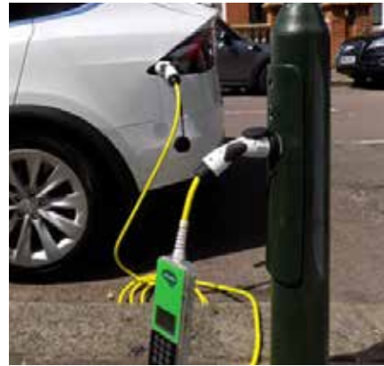
EV charging attachment to a light column. The attachment colour should match the RAL of the column
