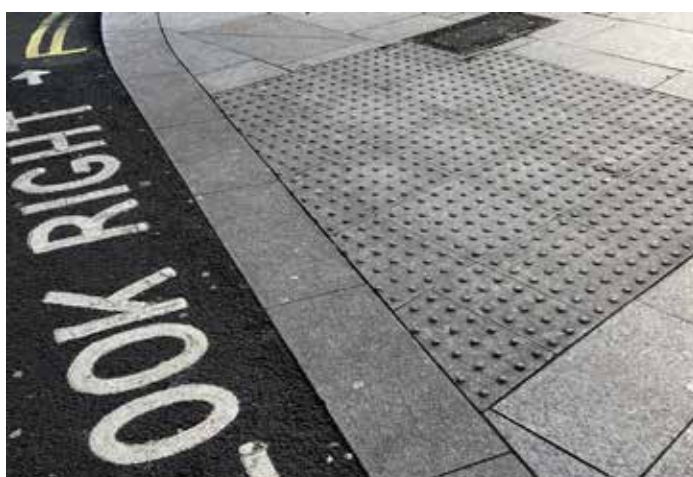
Flush kerb with tactile blister paving at uncontrolled crossing
