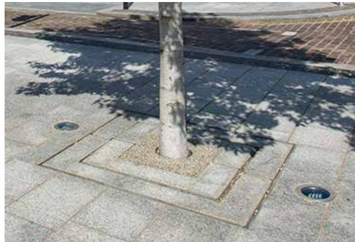
Tree grate with paving infill to match surrounding paving. The design also allows rainwater infiltration through slits and porous aggregate around the tree stem. ©GreenBlueUrban
