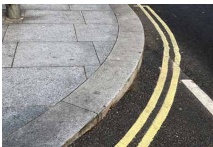
Kerb constructed using radiused kerb quadrants
