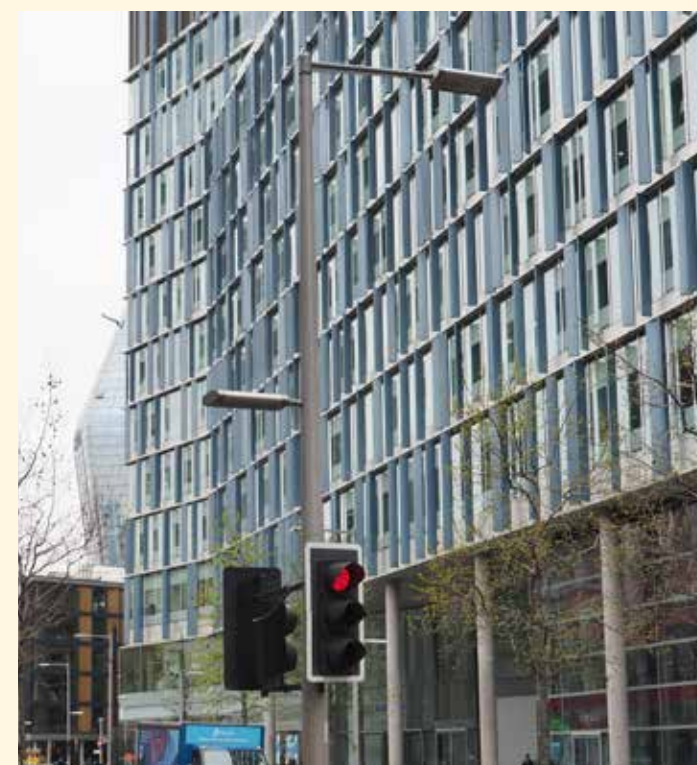
Combined lighting column with traffic signals
