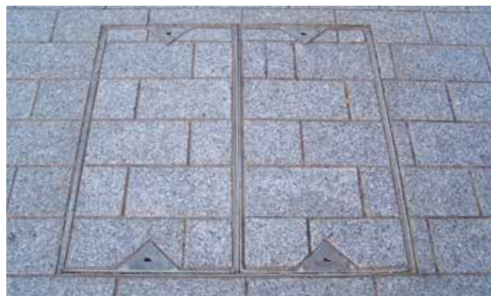
Inset utility cover with paving infill matching to surrounding paving pattern
