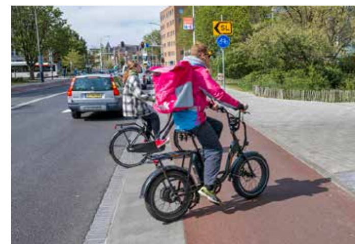
'Dutch-style' entrance kerb by Hardscape allows a cycleway/footway running across a junction to remain at a consistent level. This could be applied to both LCWIP cycle routes and vehicle crossovers for residential streets.
