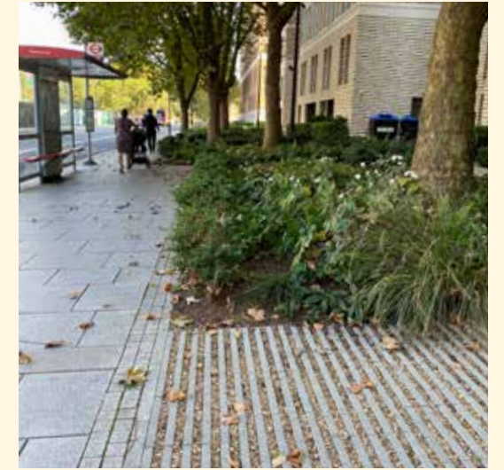
An example of permeable paving & low-level planting
