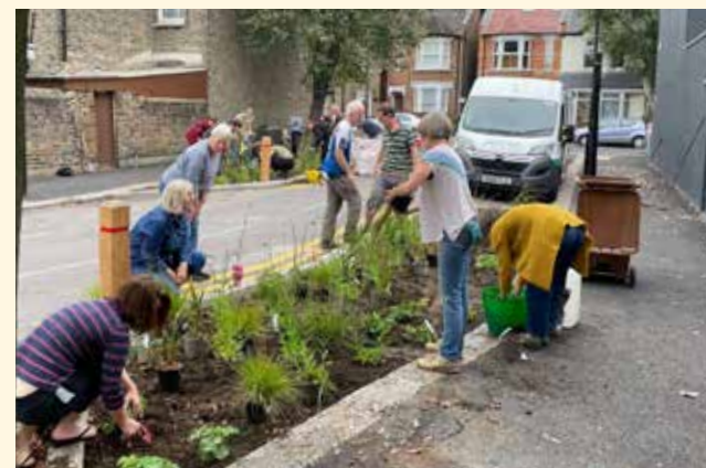
Communities could help to plant rain gardens and have a sense of ownership over planting in residential areas ©Meristem Design
